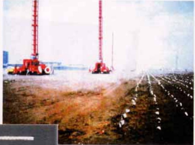
Drain Material Driving
